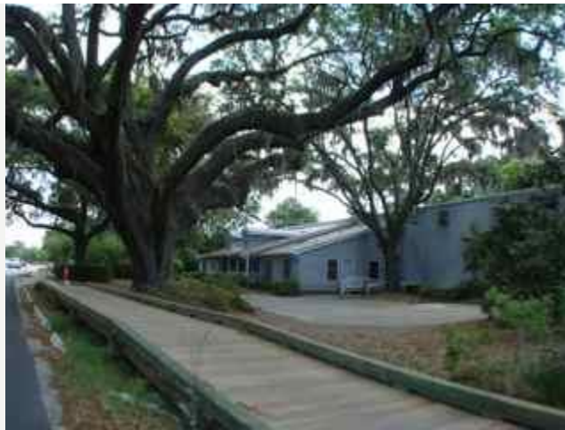
Bridging over tree roots can take many forms. This is an excellent example of a substantial bridge. But bridges do not have to be this large to protect roots. (Photo taken in Bluffton, SC)
